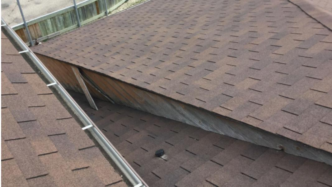
*Figure 7: New siding at gable ends adjacent to shingle elevations. Base flashings should be provided for b/w siding & shingles.*
