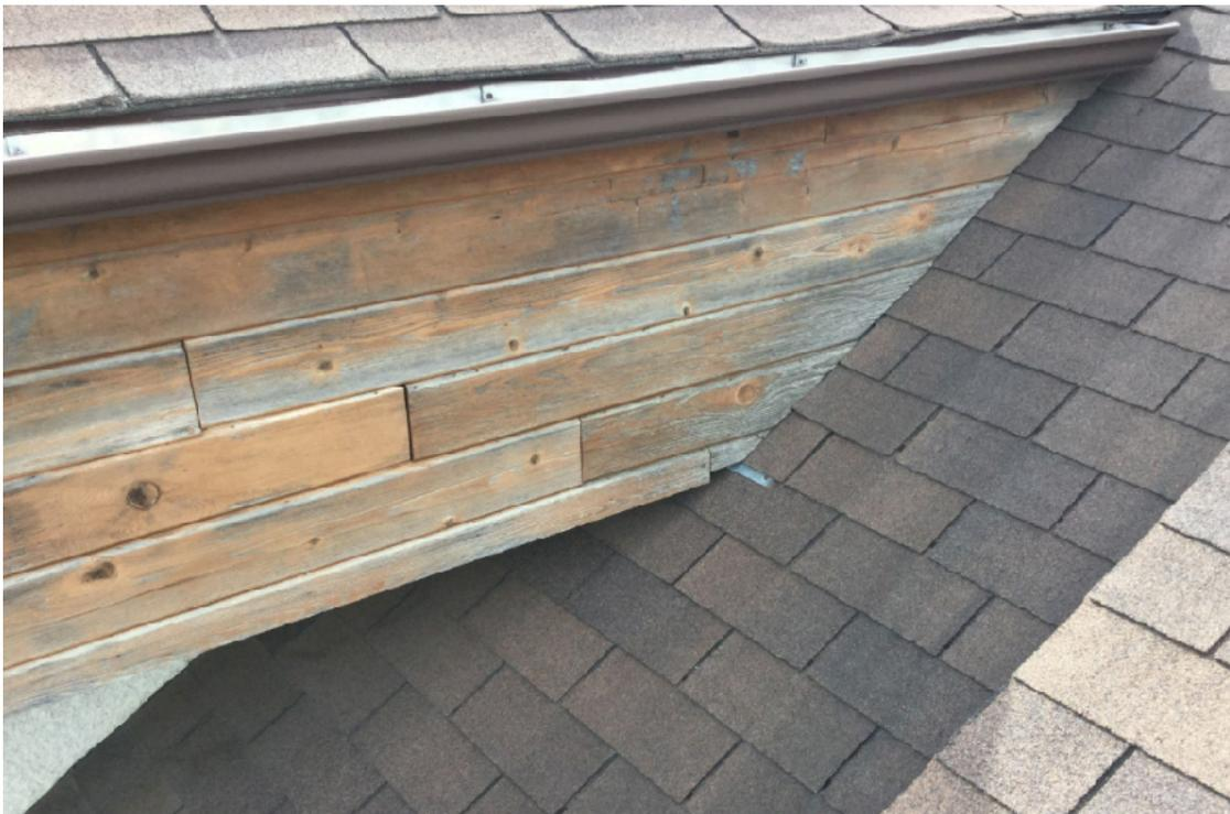
Figure 9: New siding throughout including all counter-flashings and step flashings.
