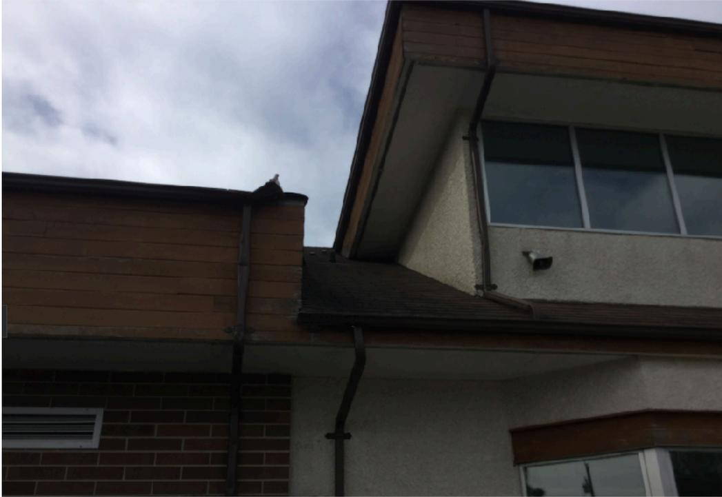
*Figure 10: Disengage and re-install down-pipes and extensions as required.*
